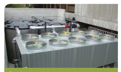
Trane reduces energy costs by incorporating an ice storage system design that uses ice made at night, when energy demand and cost are lowest, to cool the building during the day.
